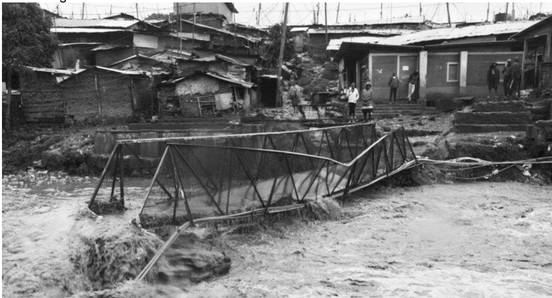
Flooding at the old KPSP05 bridge, undated
